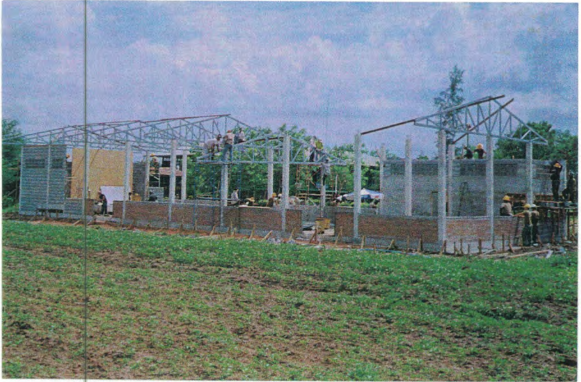
THAI AND U.S. SOLDIERS MANUALLY ERECTING THE STEEL RAFTERS
