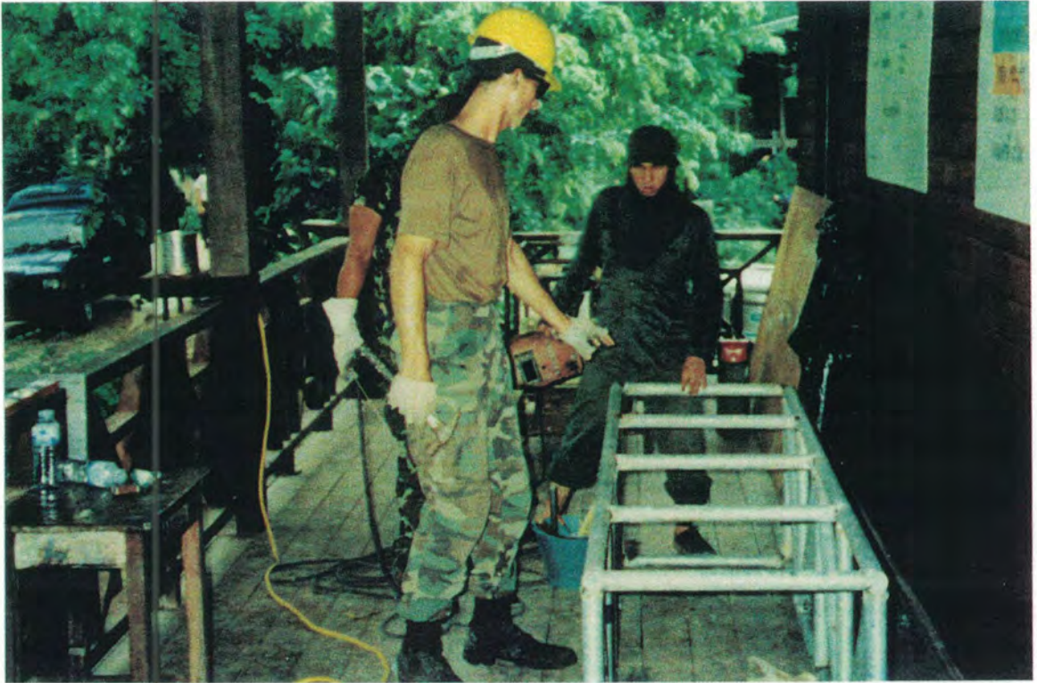
ONE OF THE THREE WELDING TEAMS PREFABRICATES A PIECE OF THE CRADLE ON THE GROUND
