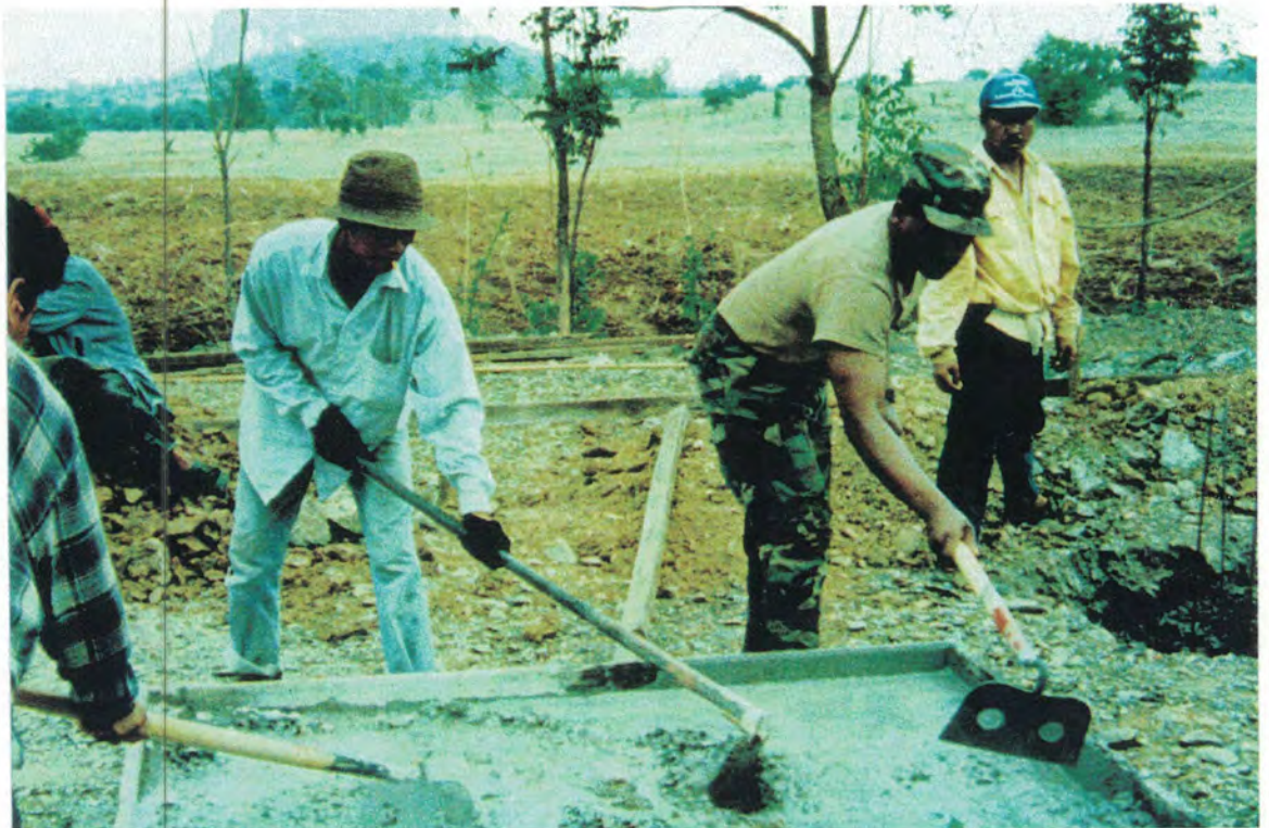
A JOINT EFFORT WAS NEEDED TO MIX THE CONCRETE BY HAND
