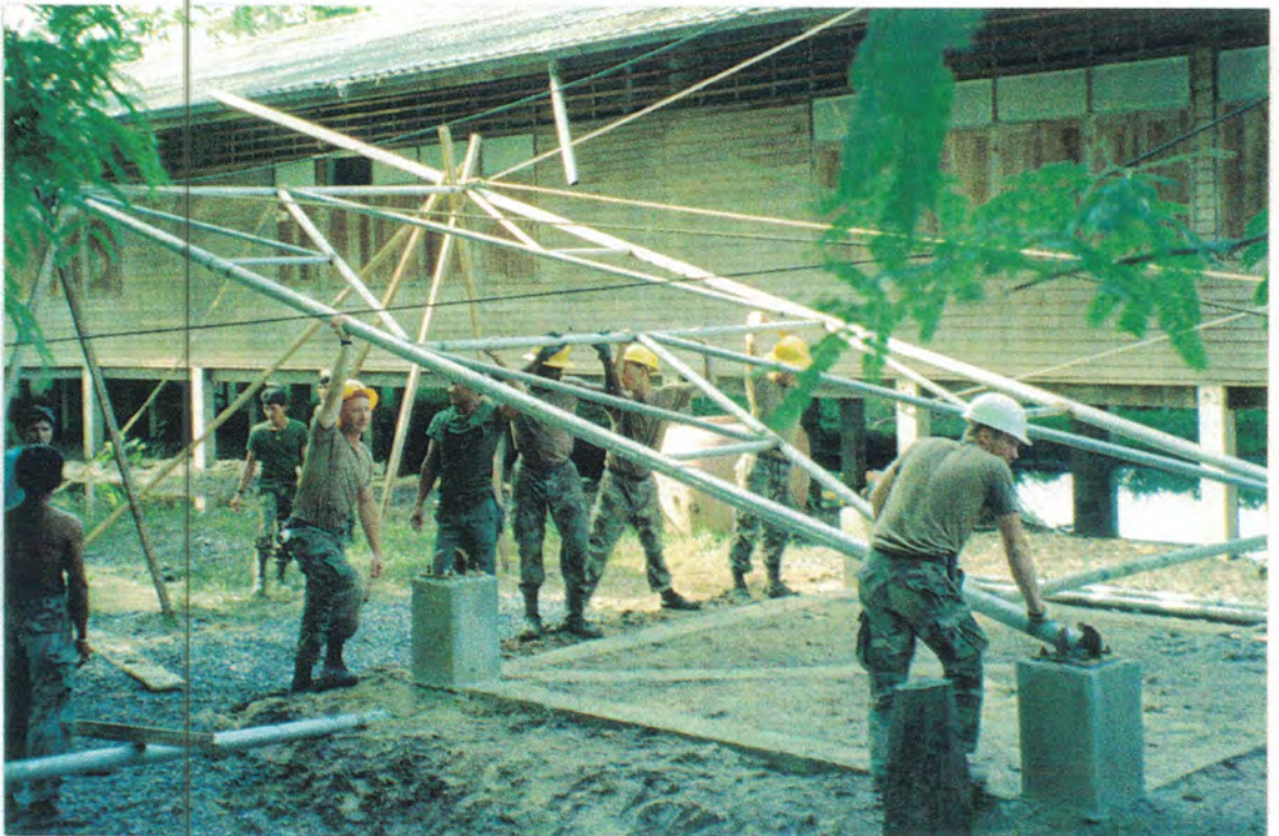
THE PREFABRICATED SIDES OF THE TOWER WERE SET UP SAFELY WITH MULTIPLE GUIDE ROPES AND 2" x 4" BRACING
