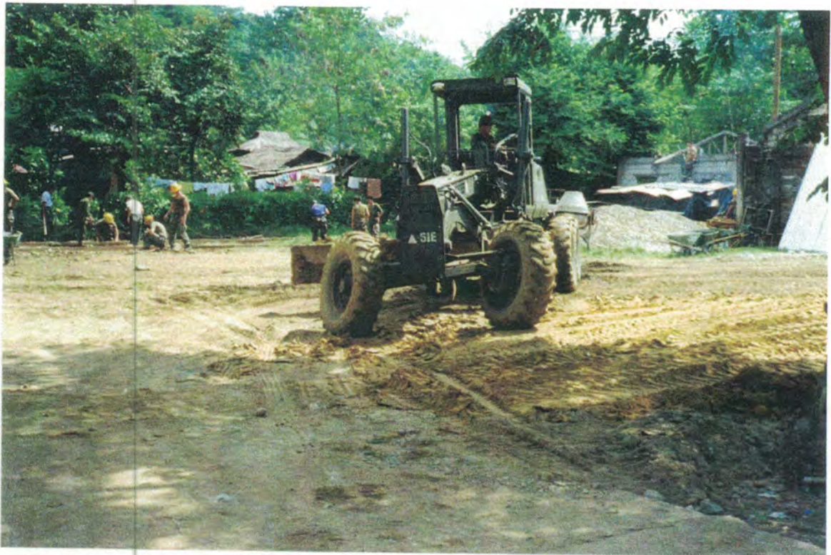
FILIPINO HEAVY EQUIPMENT OPERATOR LEVELS THE BACKFILL AS US SOLDIERS CONSTRUCT FORMWORK FOR THE FIRST 33FT X 10FT PAD.
