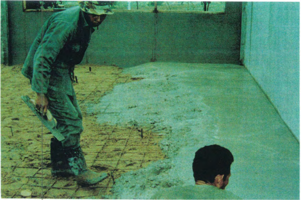
THAI 1SG DEMONSTRATES HIS METHOD OF PLACING A CONCRETE PAD
