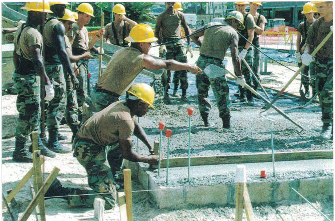
PLACING THE CONCRETE PAD
