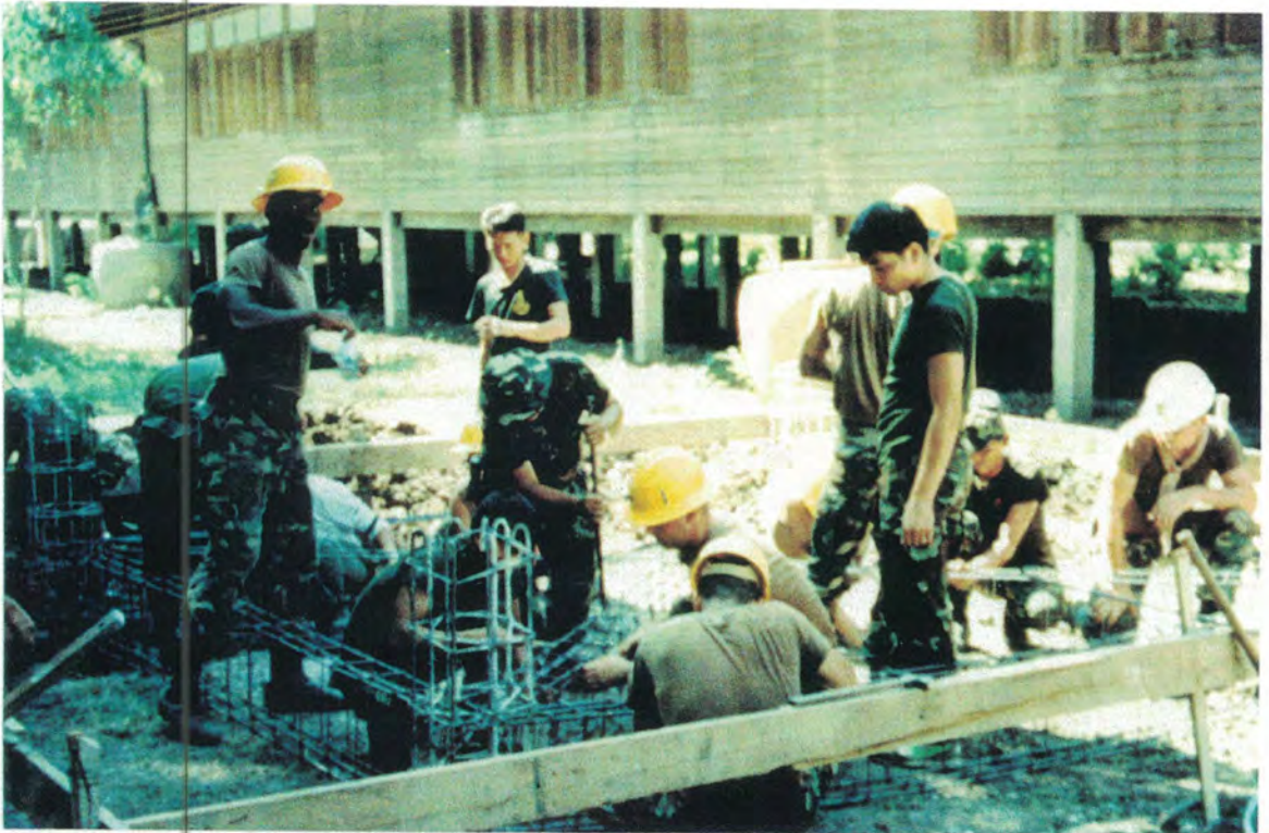
A LARGE AMOUNT OF REBAR WAS USED TO STRENGTHEN THE FOOTERS
