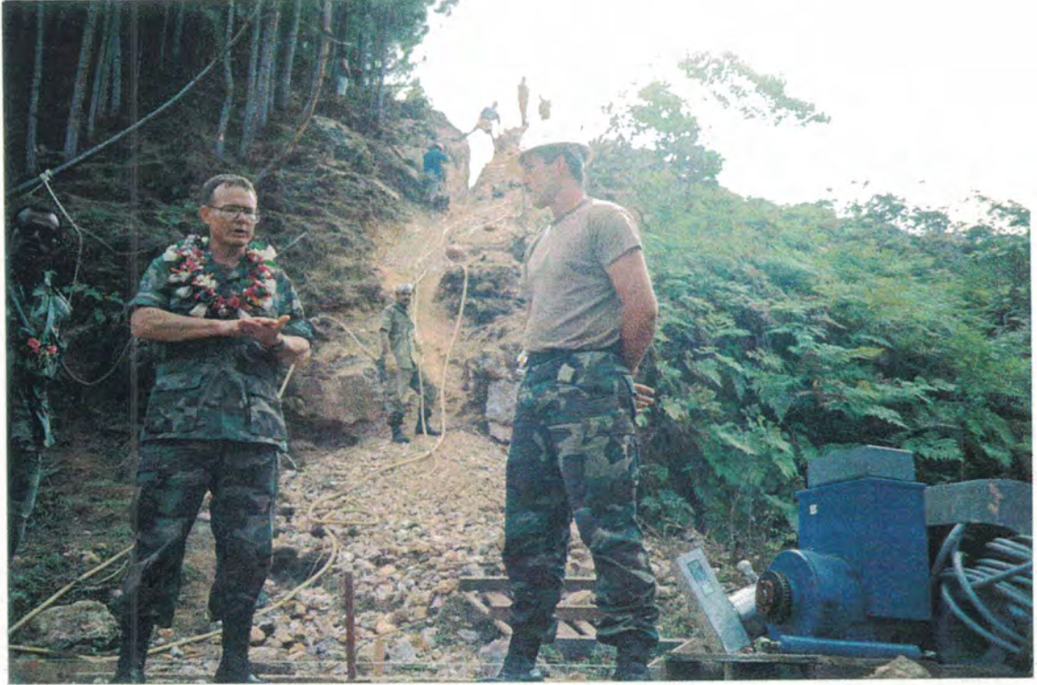
MANUALLY DIGGING THE PENSTOCK TRENCH
