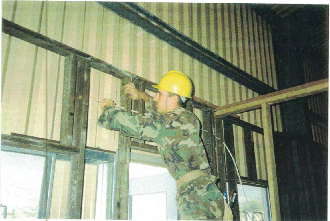
INSTALLING THE ELECTRICAL WIRE IN THE CRASH/RESCUE STATION
