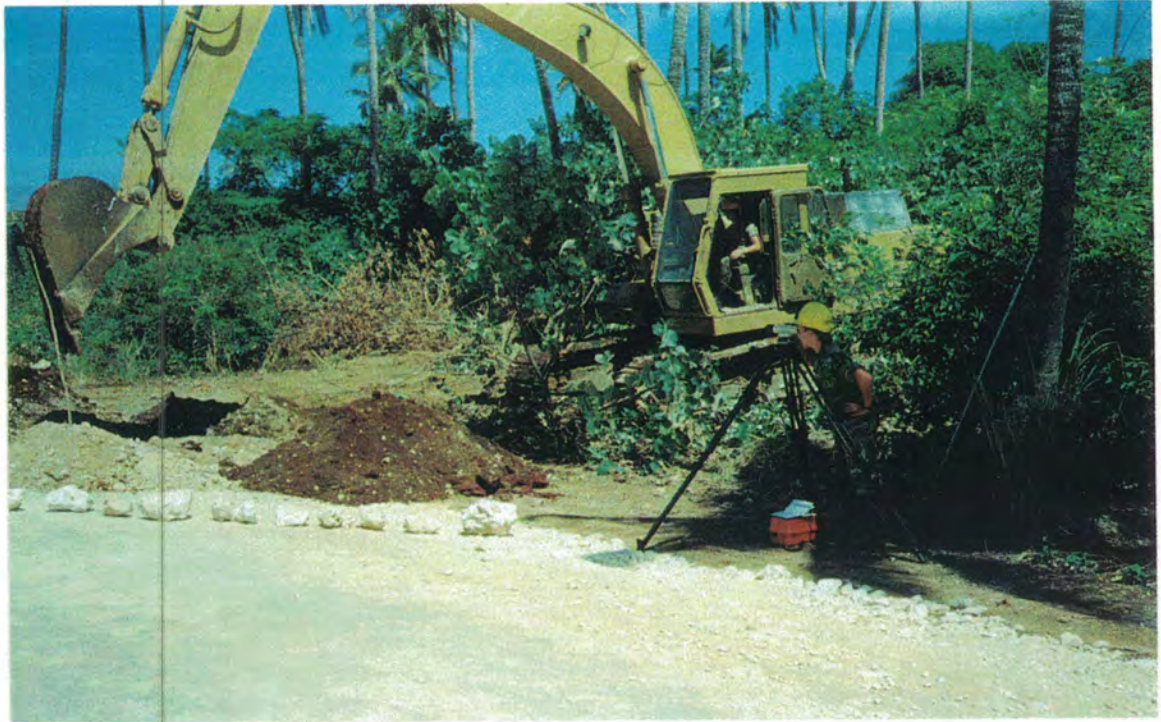
EXCAVATING FOR A CULVERT, SURVEYORS ENSURE THE PROPER GRADE IS MAINTAINED
