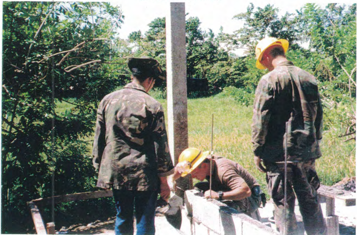
SPC DIAZ LAYS A CMU BLOCK WALL
