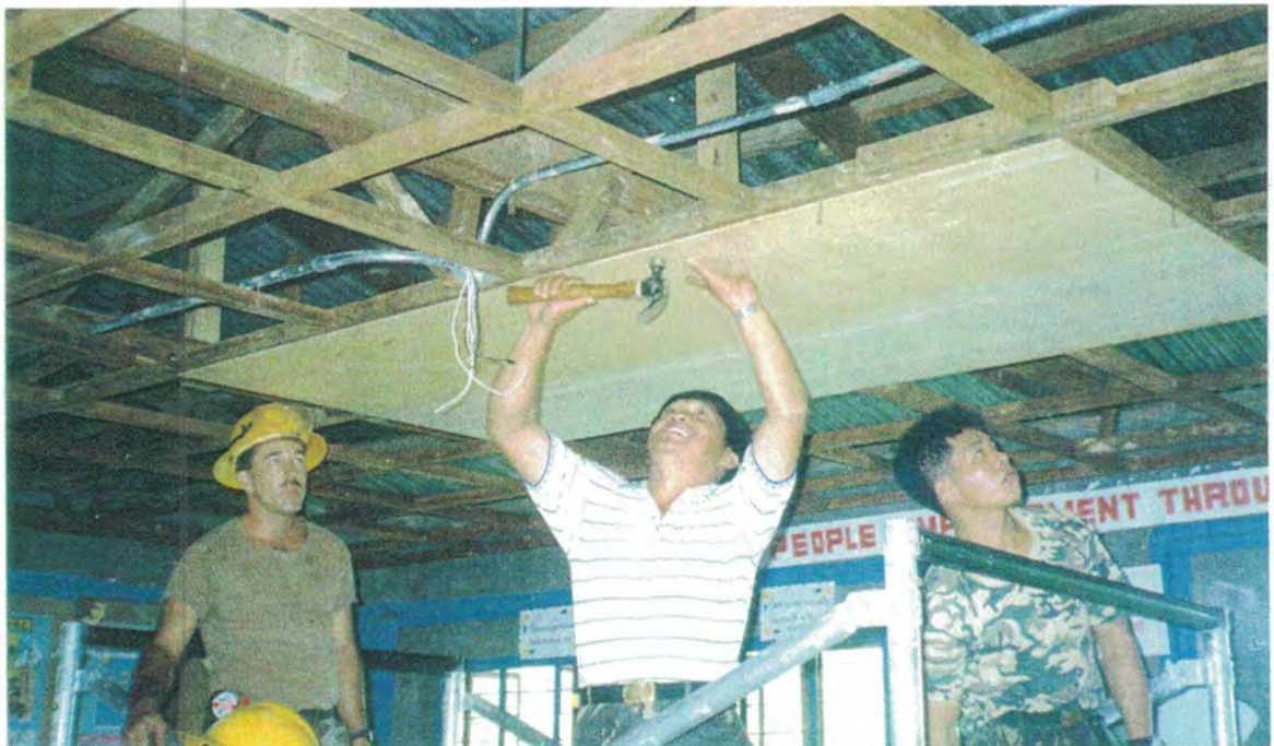
US AND FILIPINO SOLDIERS PLACE THE FIRST OF 55 SHEETS OF PLYWOOD FOR THE CEILING
