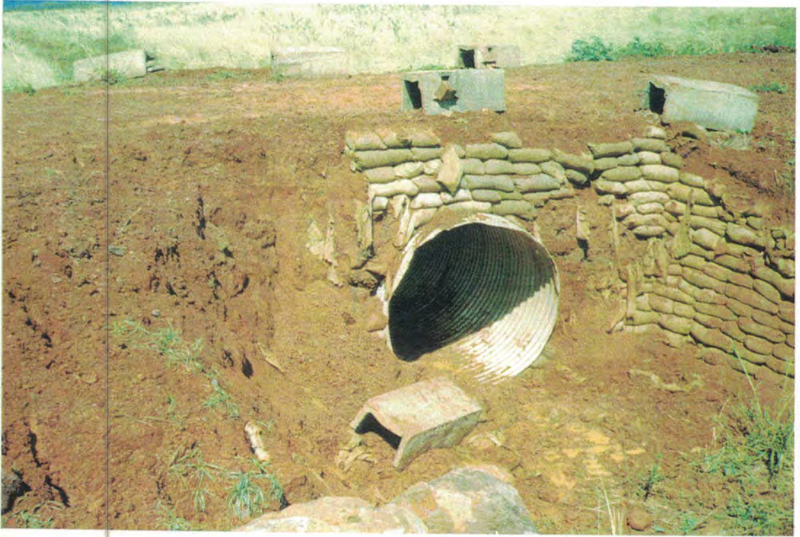
HEADWALL BEFORE, WITH AN 8 FOOT ROAD WIDTH
