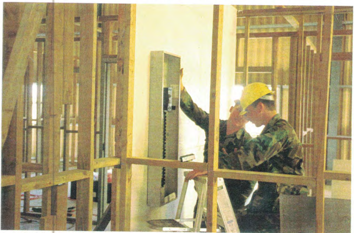
NCO TRAINING A SOLDIER TO INSTALL AN ELECTRICAL PANEL BOX
