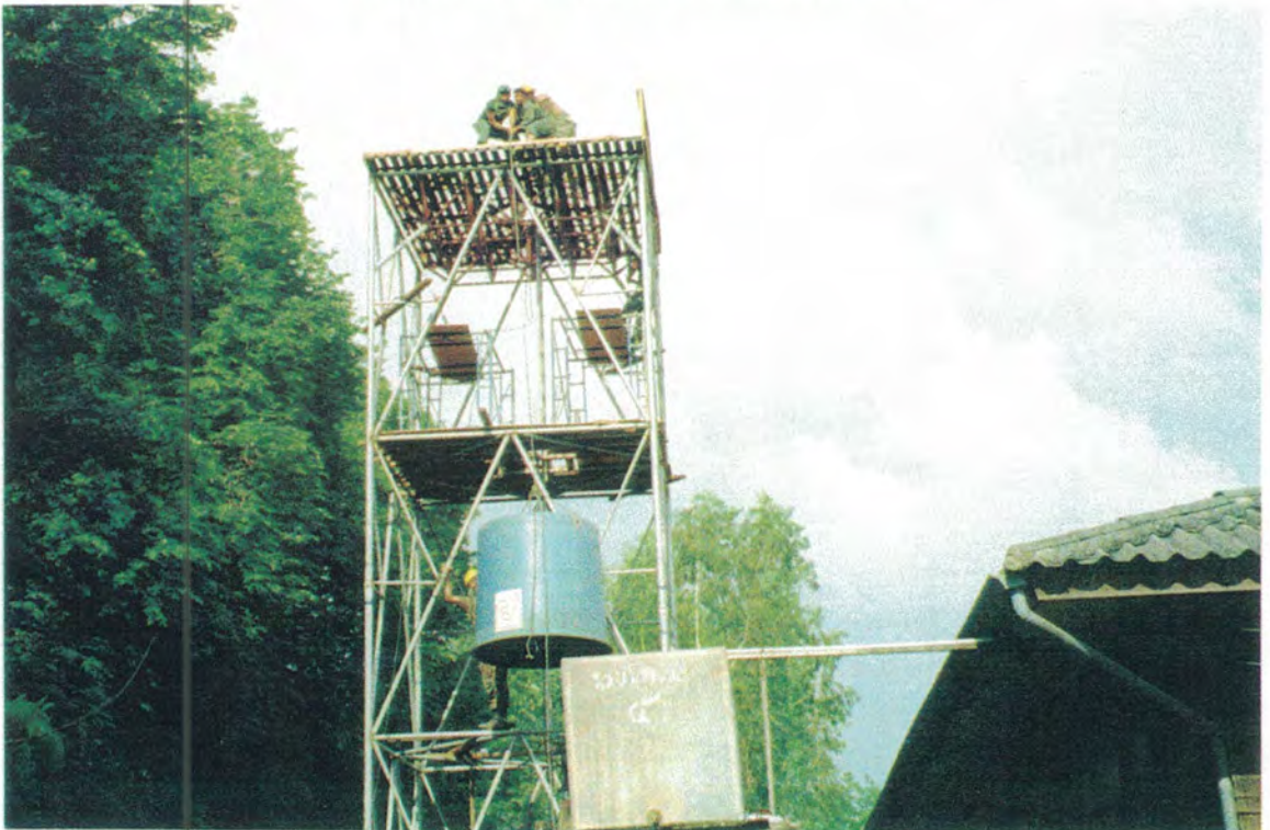
THE FIRST OF FOUR FIBERGLASS WATER TANKS IS HOISTED
