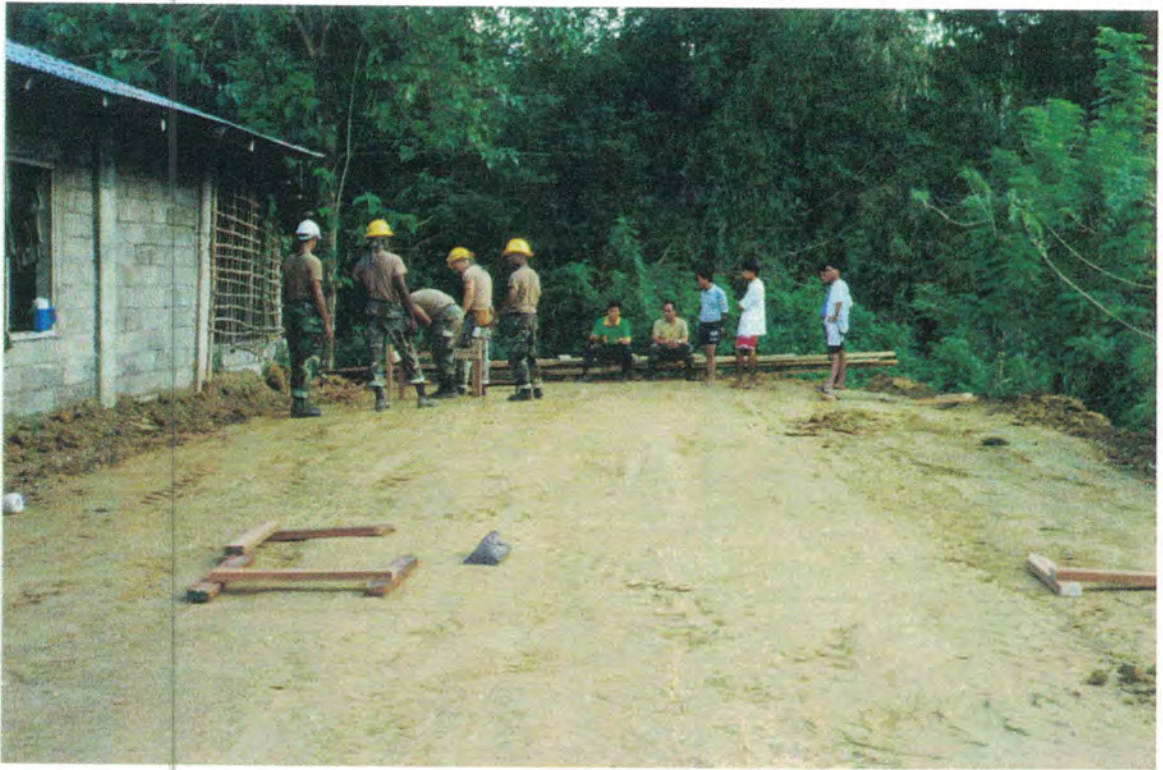
SGT PRICE'S SQUAD SETS UP THE SIGHT LAYOUT FOR THE 33FT X 16FT HEALTH CENTER
