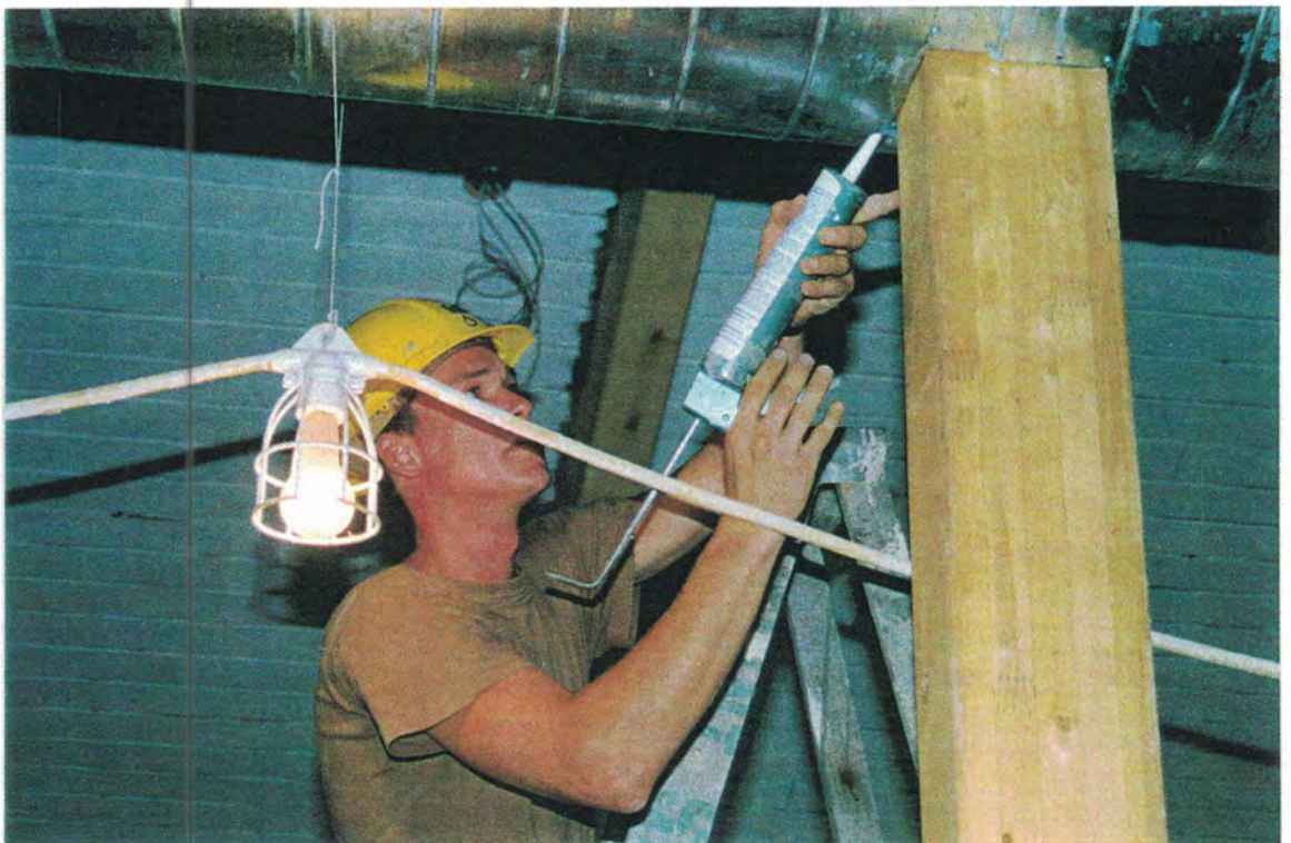
US. SOLDIER CAULKING THE AIR HANDLER DUCTWORK
