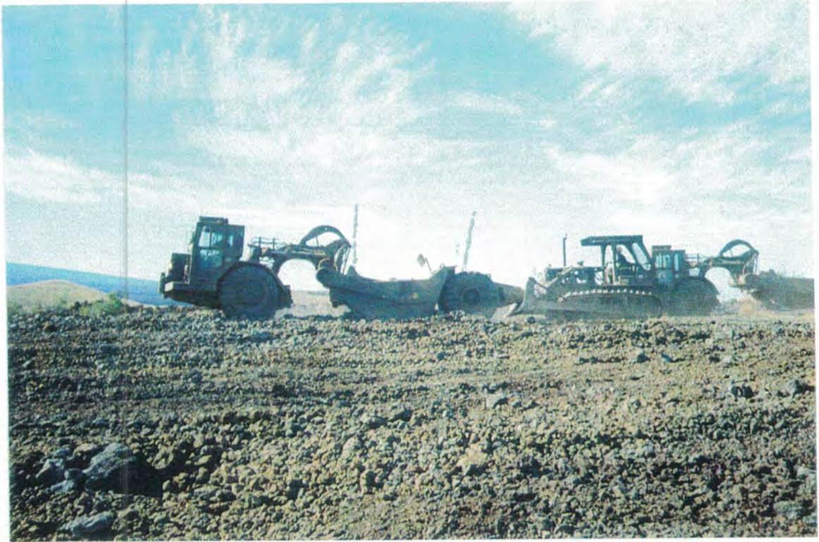
PUSH LOADING ROCK INTO SCRAPERS WITH DOZERS
