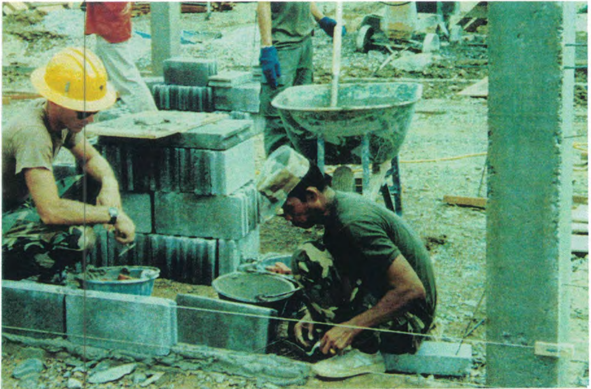
THAI AND U.S. SOLDIERS WORKING TOGETHER TO GET THE FIRST COURSE OF BLOCK STRAIGHT
