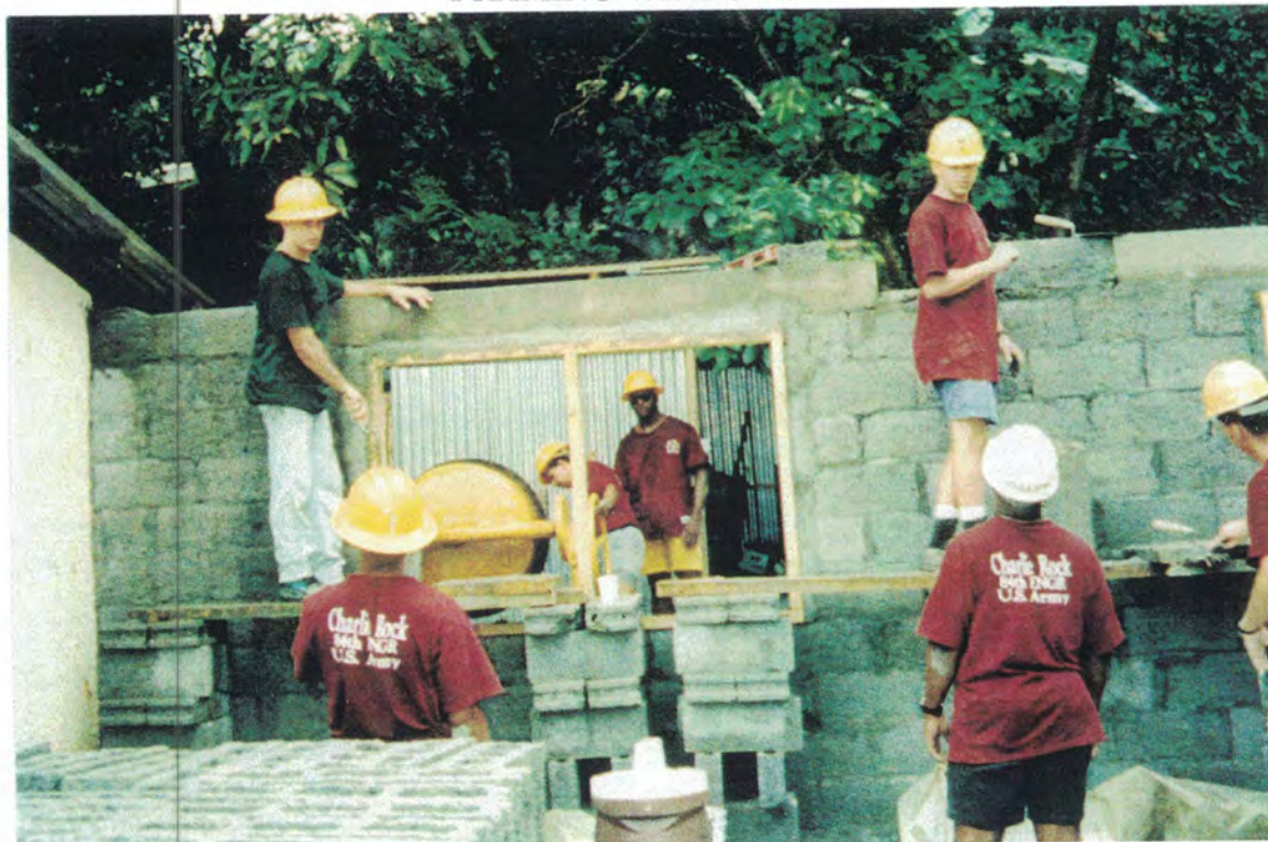
EMPLACING LINTELS
