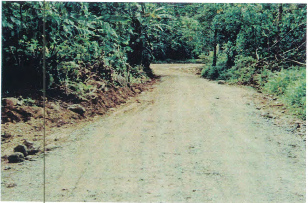
LUHOHK ROAD COMPLETED, 4M TRAVEL WAY x 1500M LENGTH
