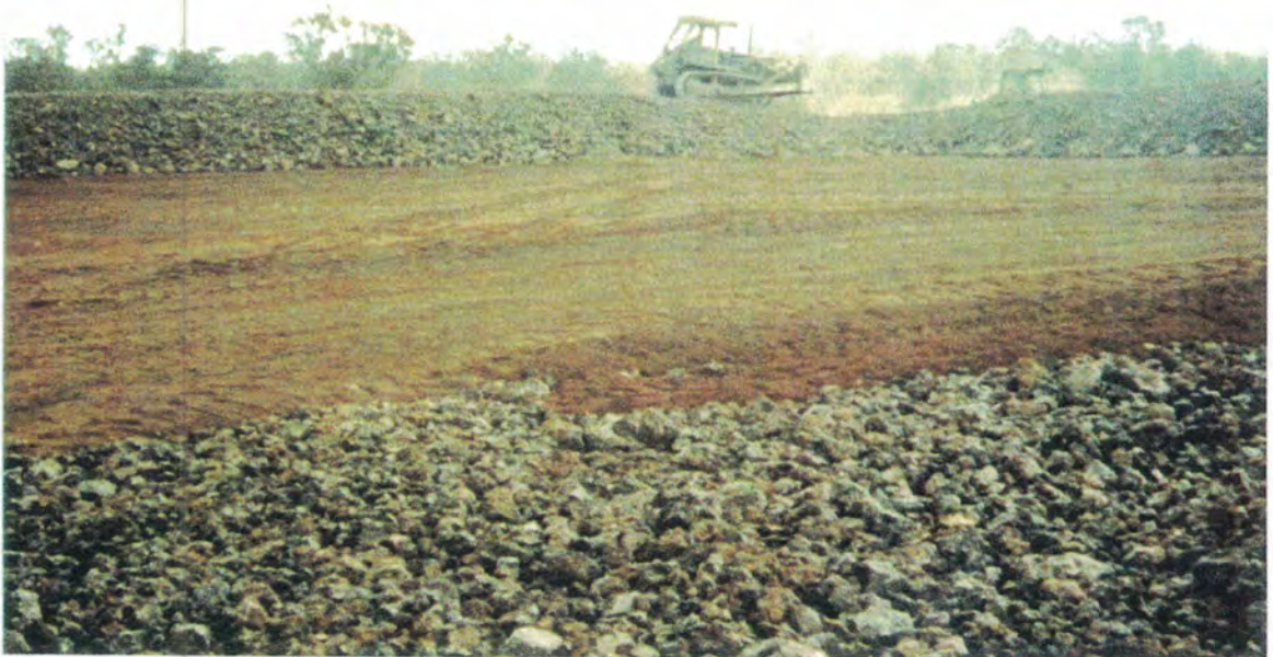
DOZER COMPACTING THE BERMS OF FOWARD AREA AMMUNITION AND REFUELING POINT STORAGE AREA IN LAVA FIELD
