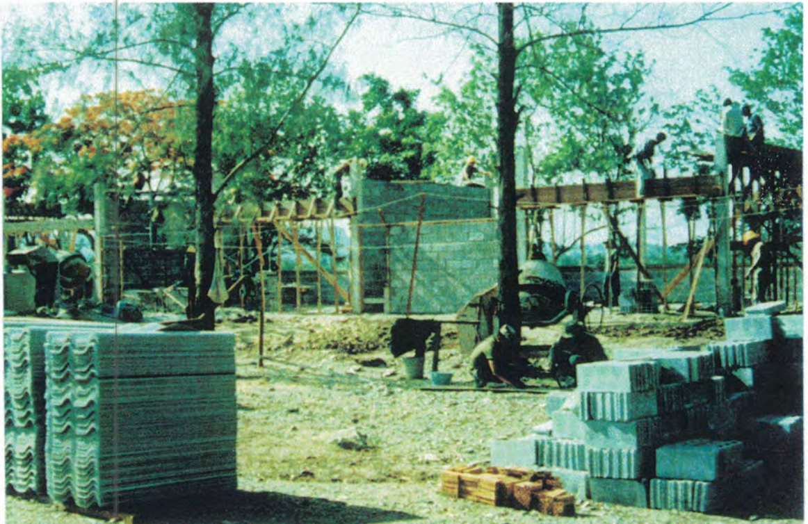
CONSTRUCTION OF FORMWORK FOR THE HORIZONTAL COLUMNS
