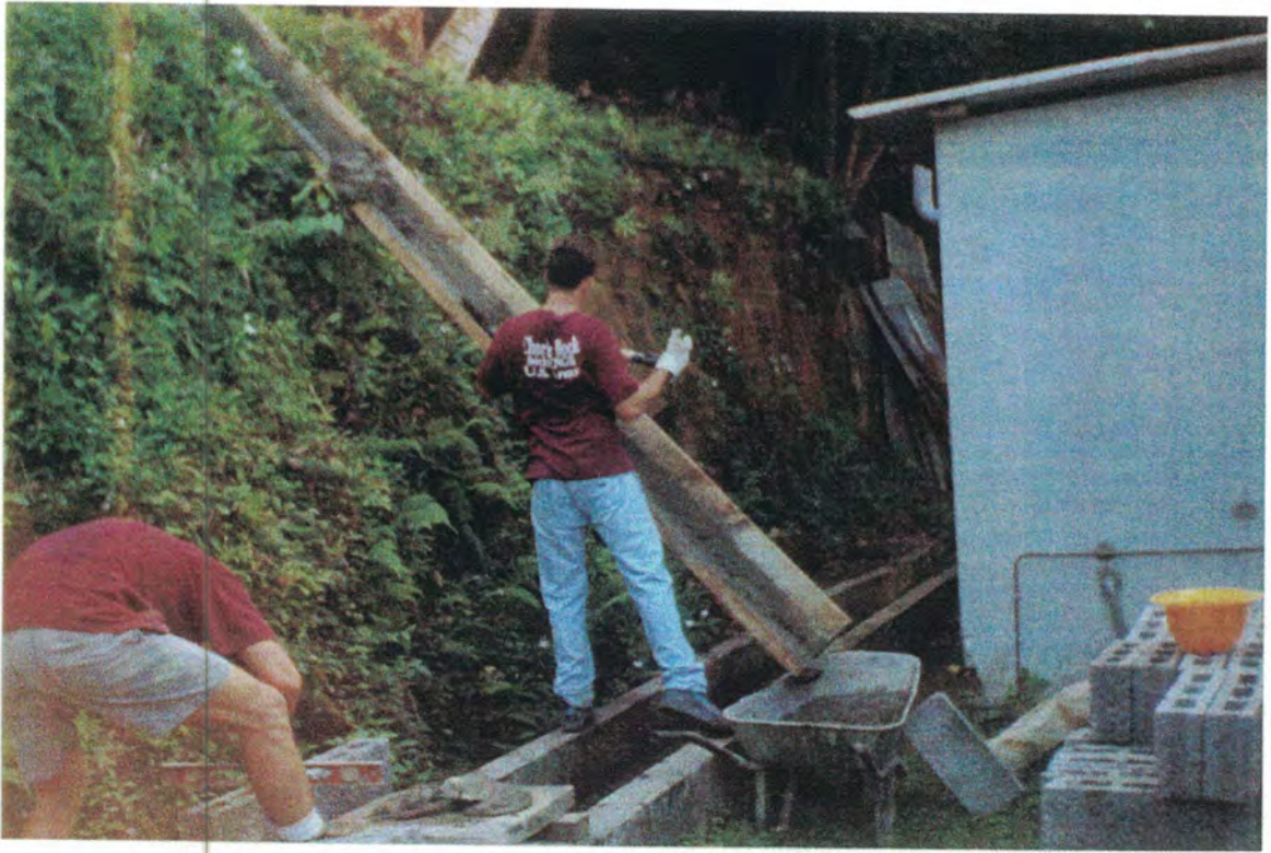
MORTAR AND BLOCK CHUTE FOR BUILDING RETAINING WALL
