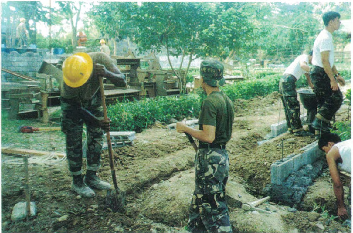
PFC WOODS ASSISTS THE FILIPINO SOLDIERS IN EXCAVATING THE GROUND FOR THE SIDEWALK AND DRAINAGE DITCH
