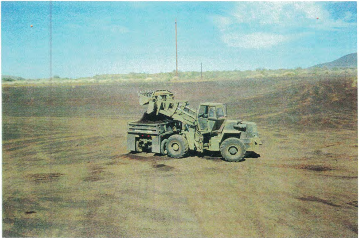
LOADING A 5 TON DUMP TRUCK AT BORROW PIT
