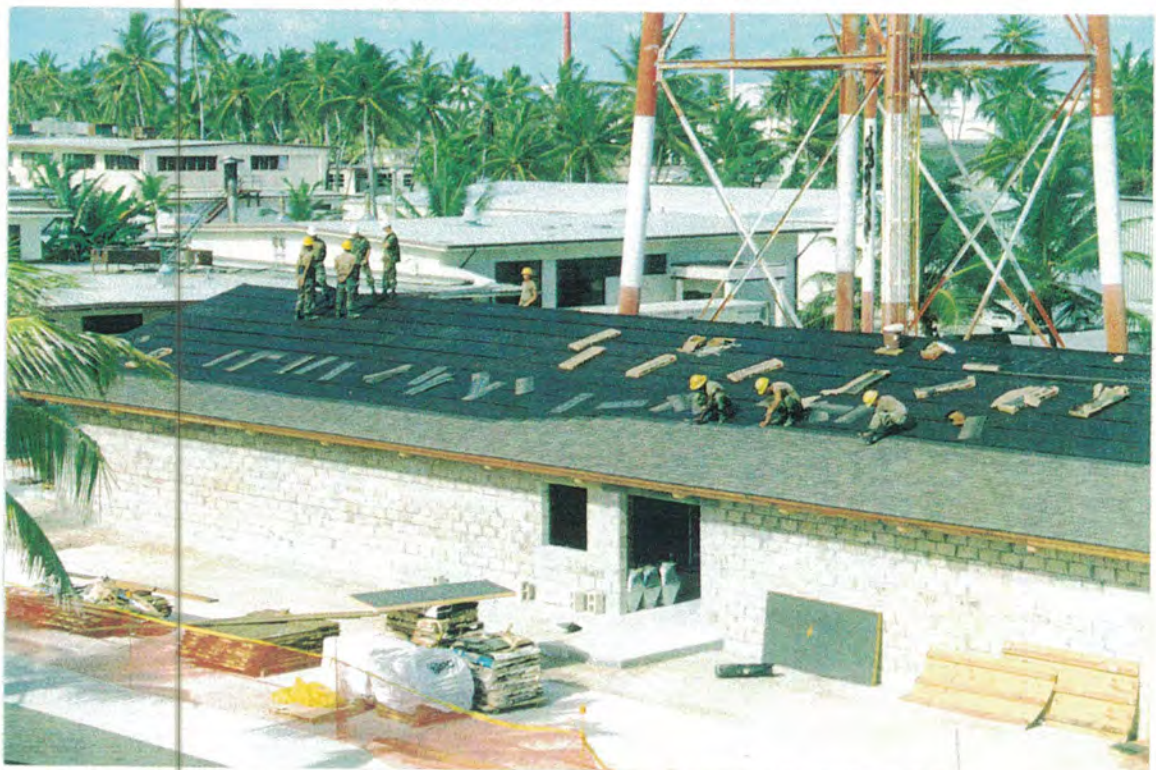
U.S. SOLDIERS WORK AT SHINGLING THE ROOF
