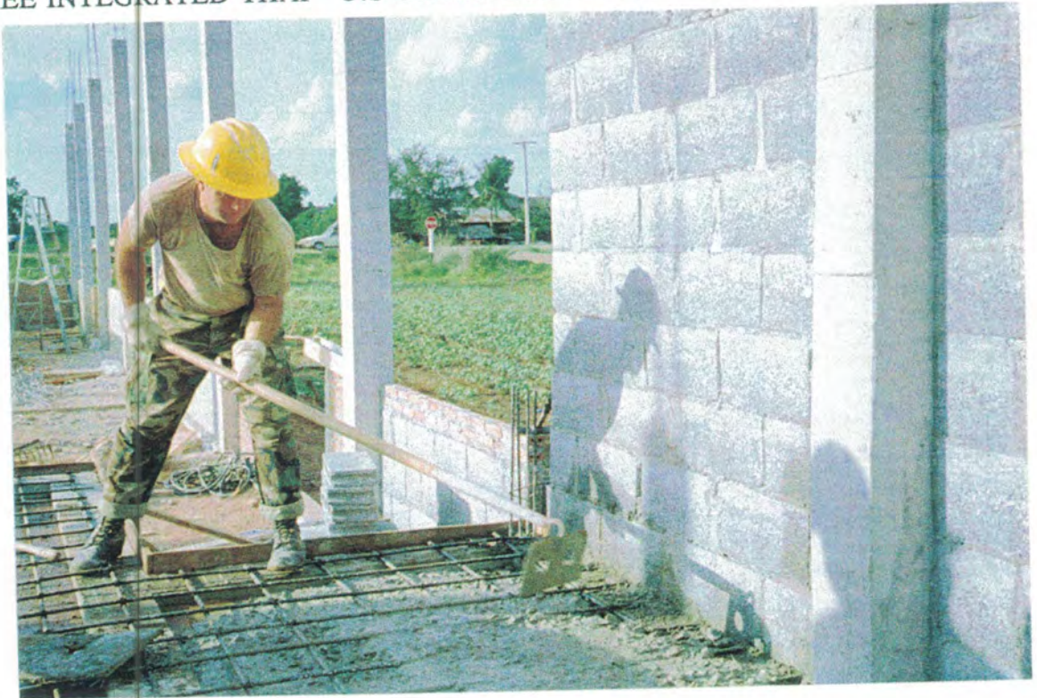
PLACING CONCRETE FOR STAGE IN FRONT OF THE AUDITORIUM
