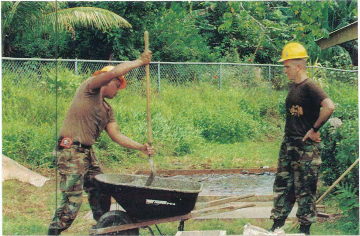
MIXING & PLACING CONCRETE FOR WATER CATCHMENT PADS
