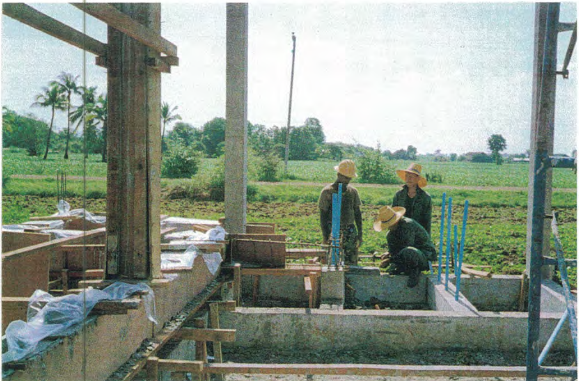
U.S. AND THAI SOLDIERS REMOVING THE ELABORATE FORMWORK
