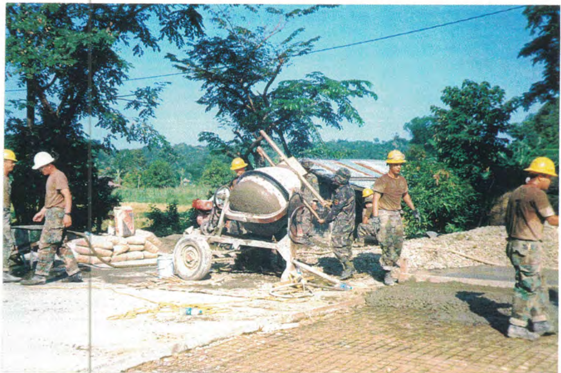
JOINT EFFORT MIXING AND PLACING CONCRETE
