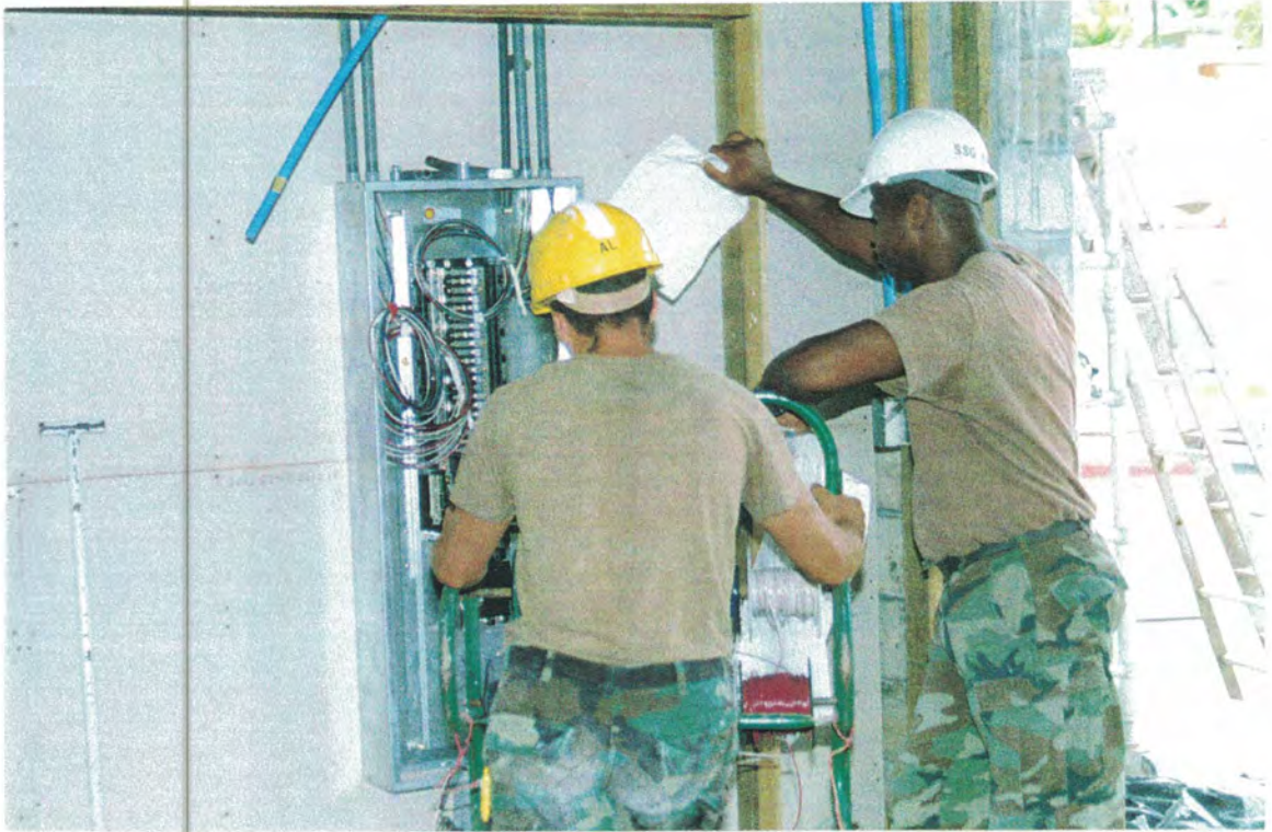
INSTALLATION OF THE THREE PHASE ELECTRICAL SYSTEM
