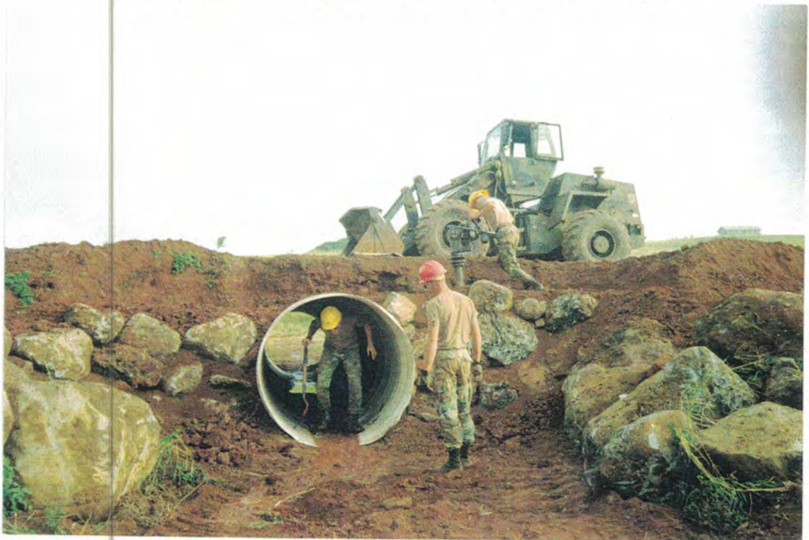
4" TO 6" LIFTS WERE HAND COMPACTED AROUND THE CULVERT
