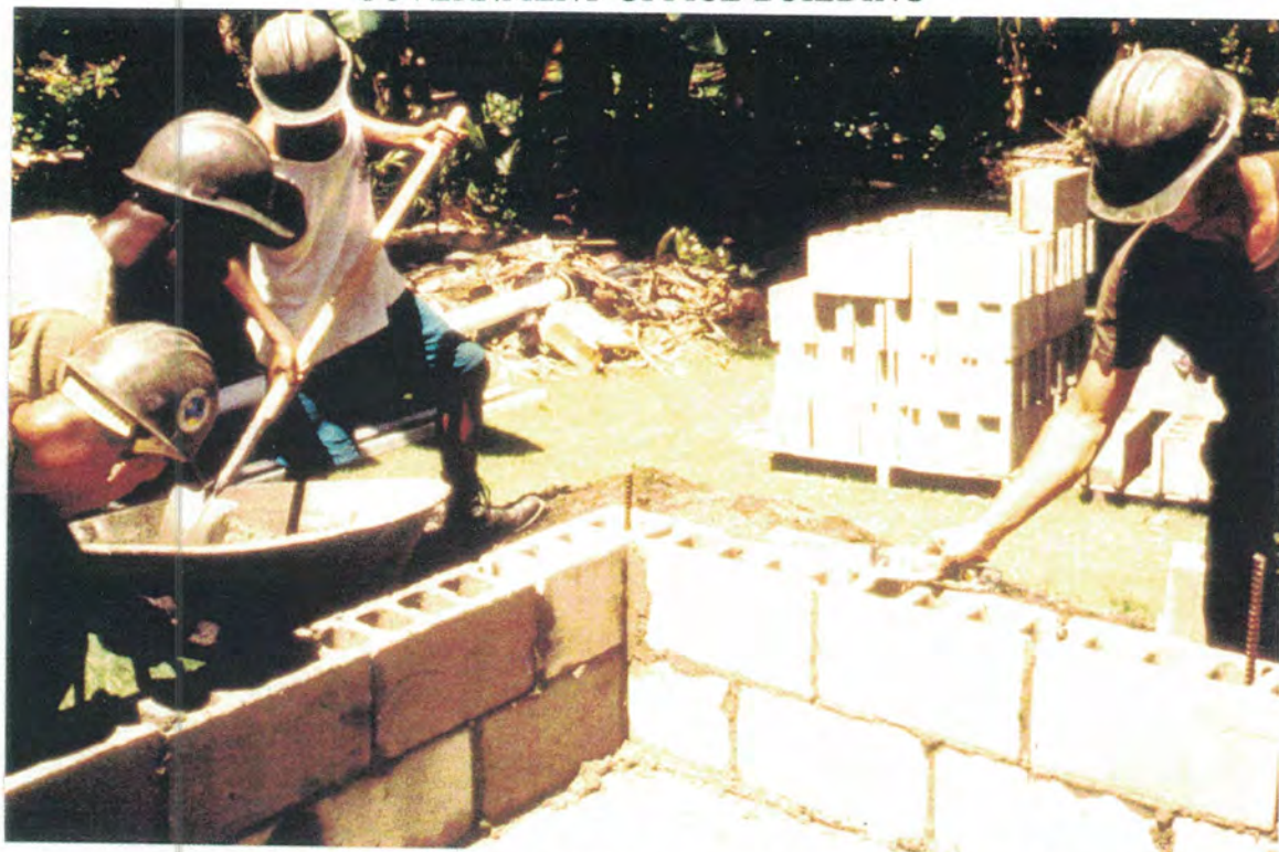
LAYING BLOCK WHILE CONSTRUCTING A FEMALE LATRINE
