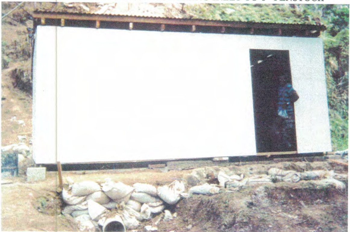
TURBINE SHED - NOTE 8" OUTLET
