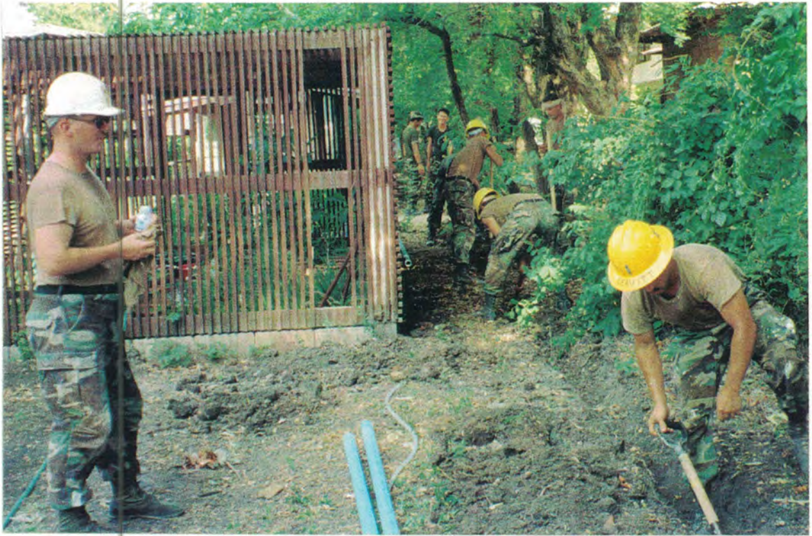
A QUARTER MILE OF PIPE IS INSTALLED CONNECTING THE SCHOOL FACILITIES AND THE WATER TOWER
