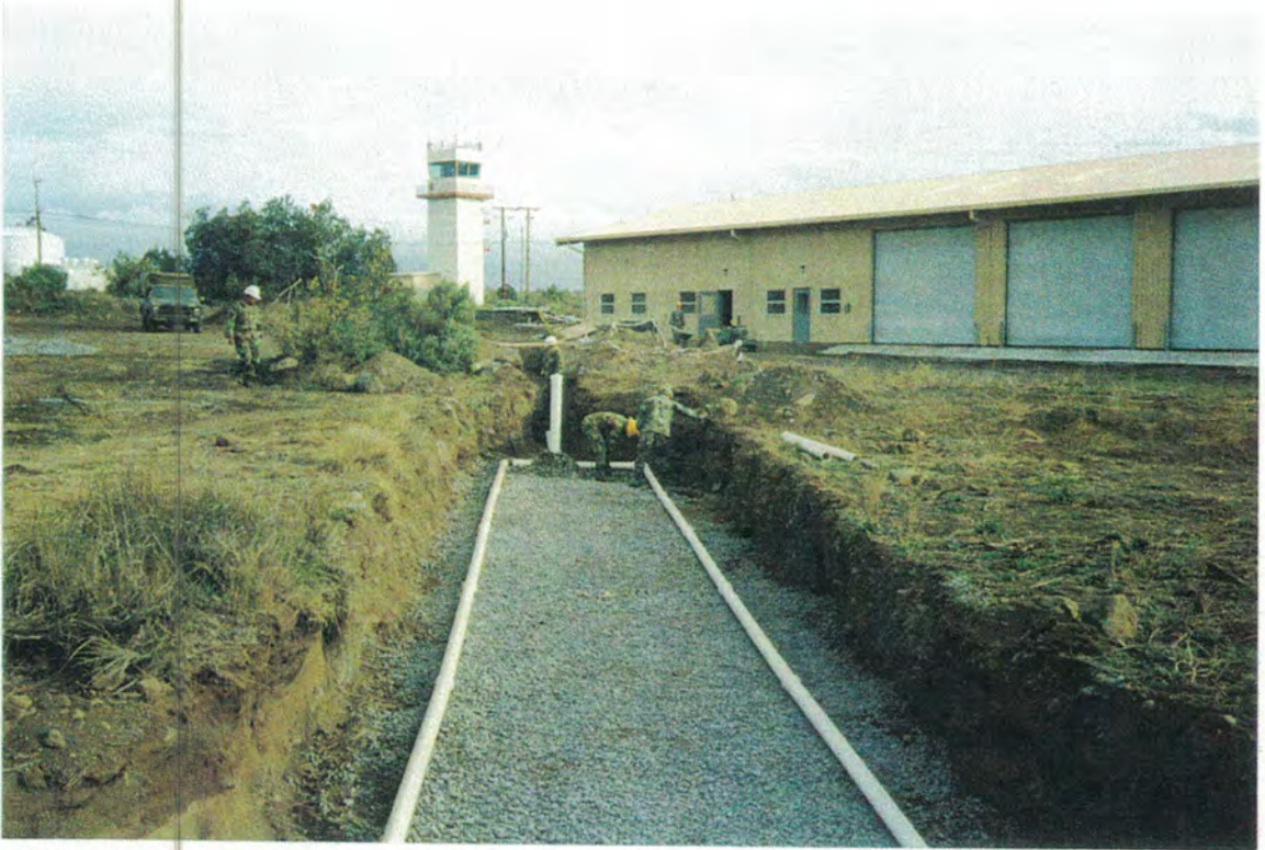
WORKING TO GET THE CORRECT SLOPE ON THE 48 FOOT LONG LEACH FIELD
