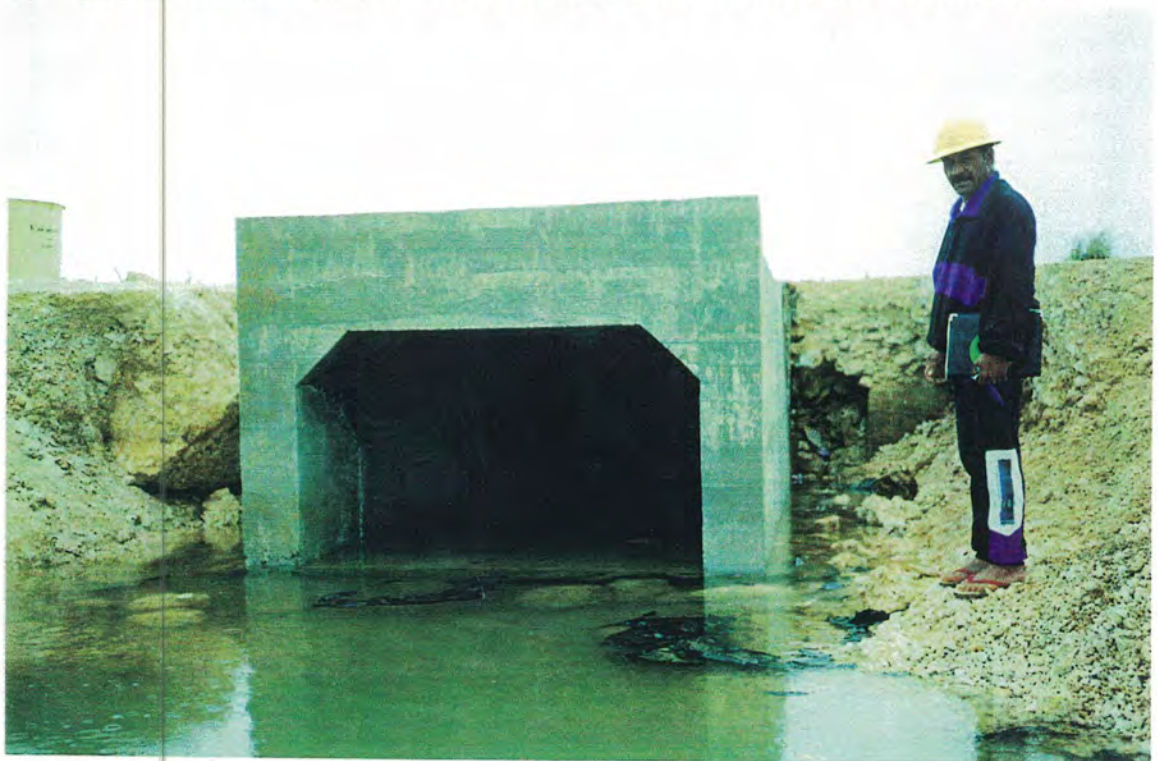
COMPLETED 16'x10'x6' CULVERT
