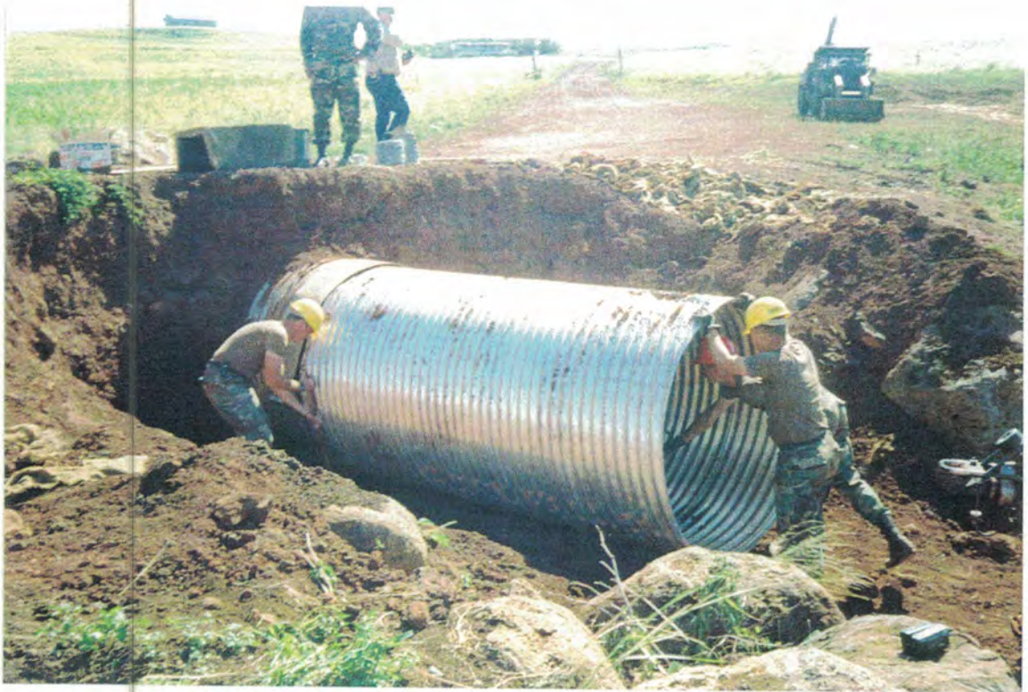
PLACING THE 10 FOOT SECTION OF 60" CULVERT
