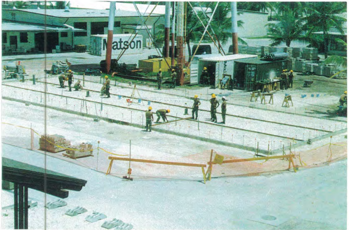
PLACING FORMWORK FOR 103' X 38' CONCRETE PAD
