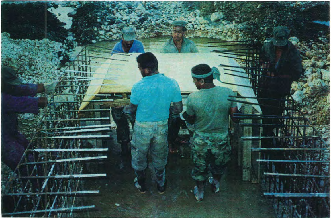
TDS SOLDIERS PLACE FORMWORK FOR A CAUSEWAY CULVERT
