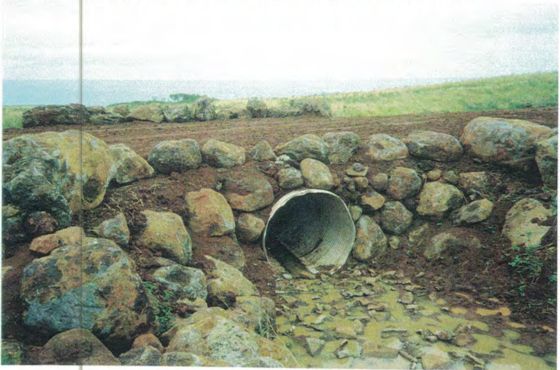
HEADWALL AFTER, WITH A 15 FOOT ROAD WIDTH
