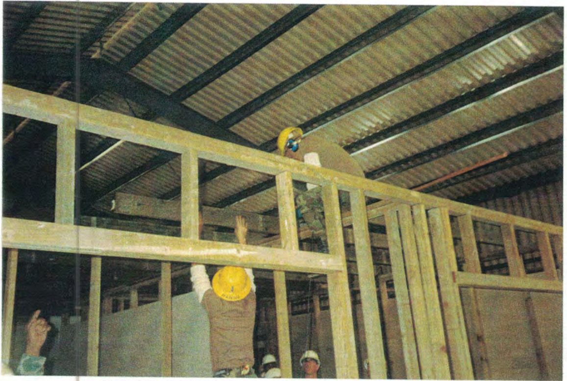
CARPENTERS INSTALLING THE CEILING JOISTS
