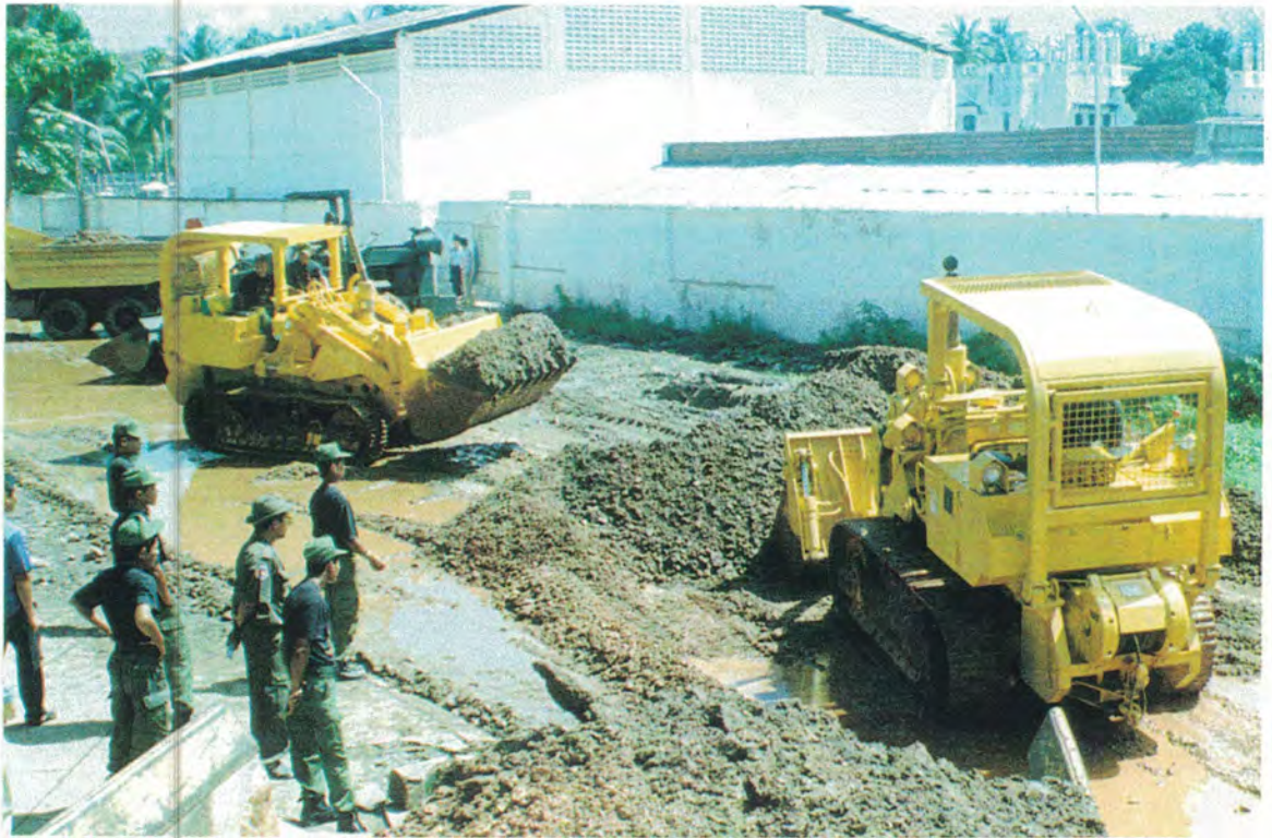
RCAF SOLDIERS USE TWO TRACKED SCOOP LOADERS IN UNISON TO REMOVE A STOCKPILE
