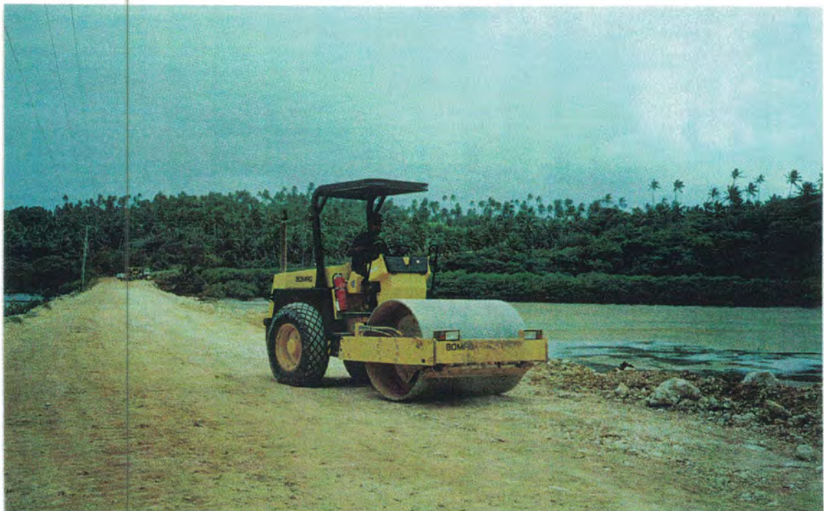
NEWLY TRAINED TDS SOLDIER COMPACTS CAUSEWAY ON A VIBRATORY ROLLER
