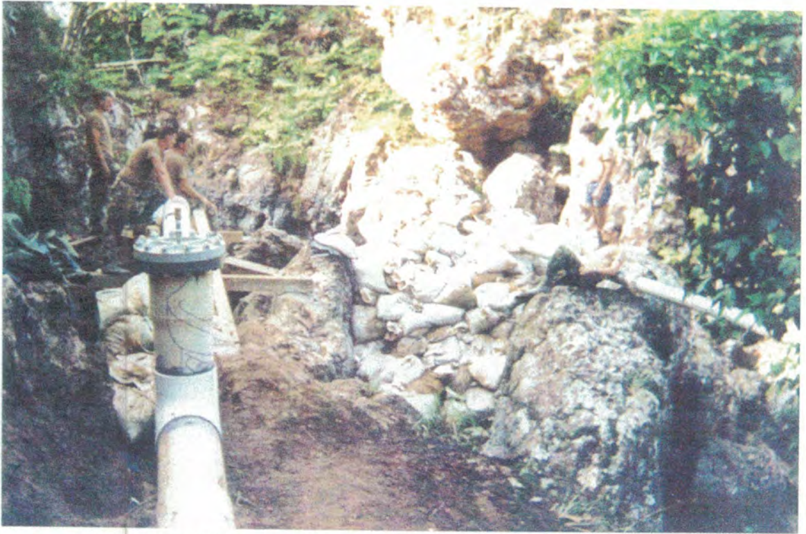
DAMMING STREAM AND INSTALLING INLET TO 8" PENSTOCK
